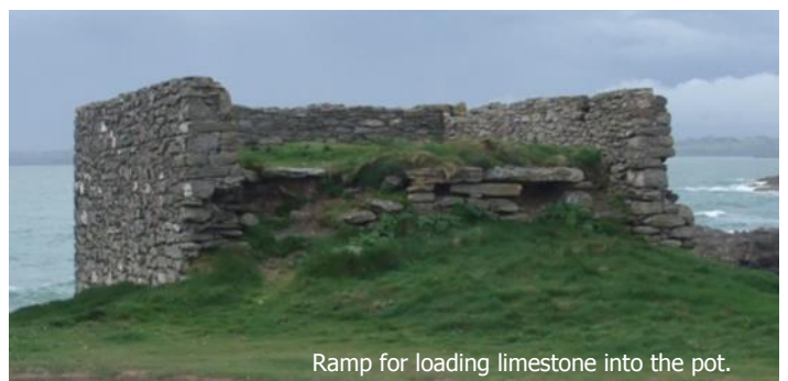
The pot is lined with blocks of Old Red Sandstone.
