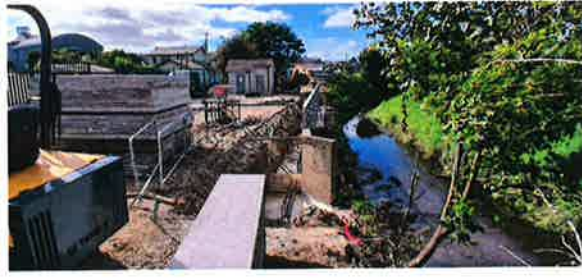
Construction of RC Retaining Wall
