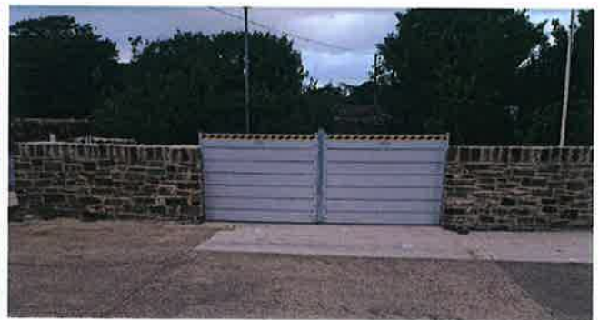
Installation of a demountable flood defense wall
