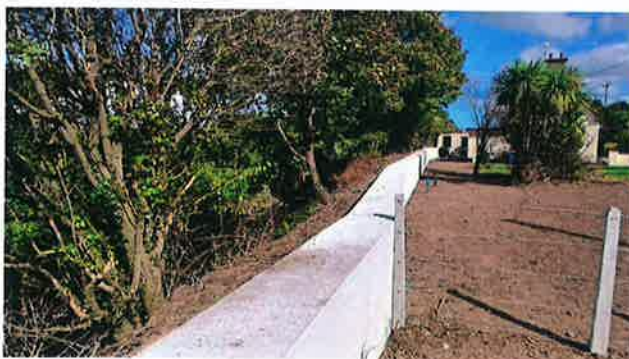
Completed flood retaining wall
