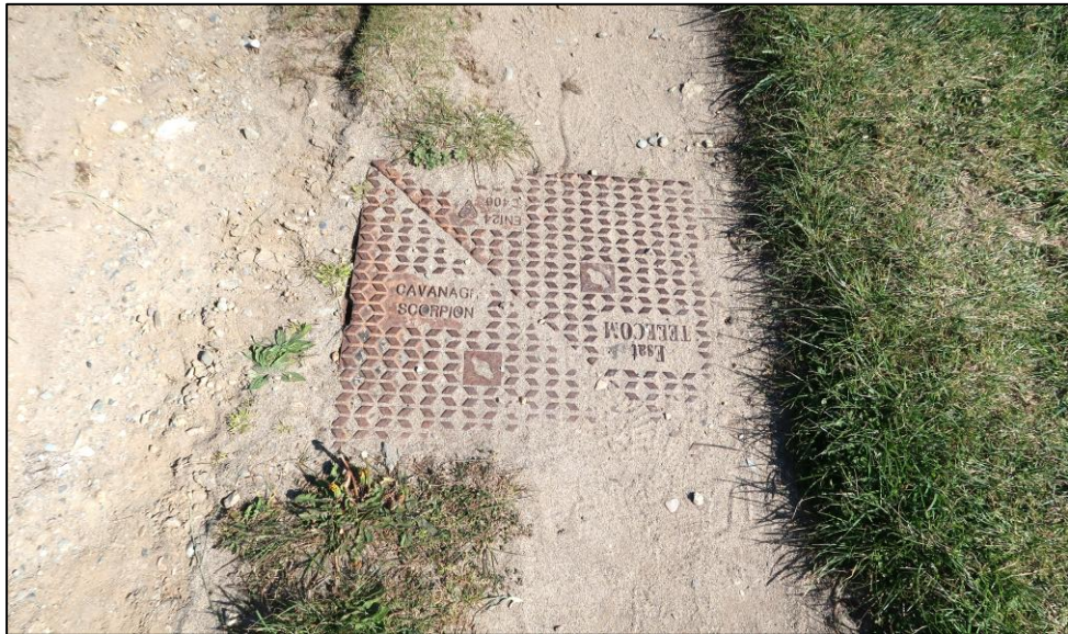
Plate 17. Metal manhole cover.
