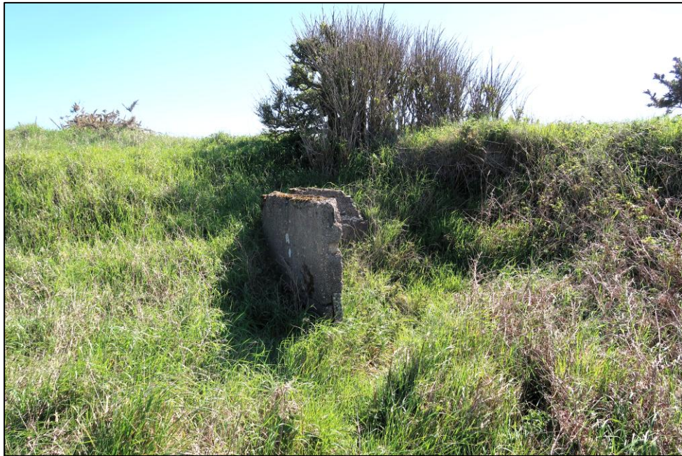
Plate 20. Ruined remains of cased concrete walls.
